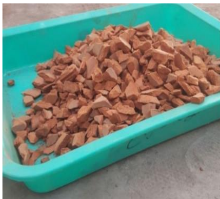
Fig1. Broken roof tile
