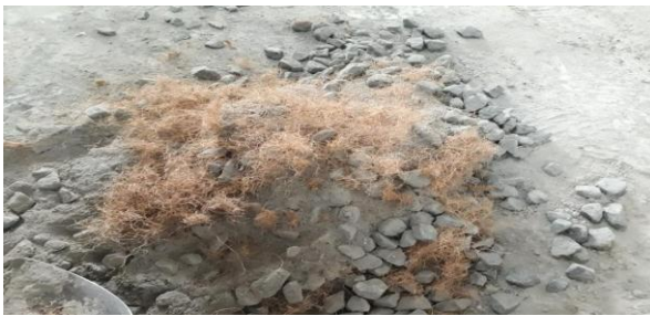
Mixing of concrete
