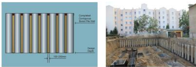
(Fig 15. Contiguous pile wall in basement constructions)
