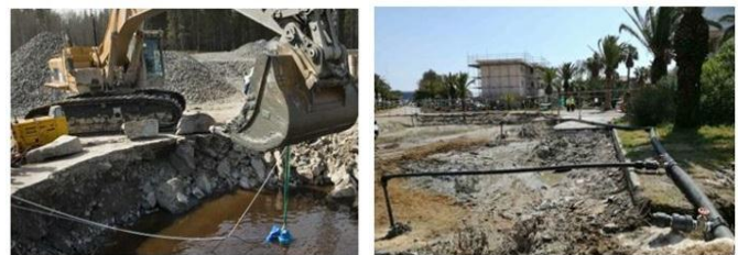
(Fig 1.Sump pumping and deep well points)
