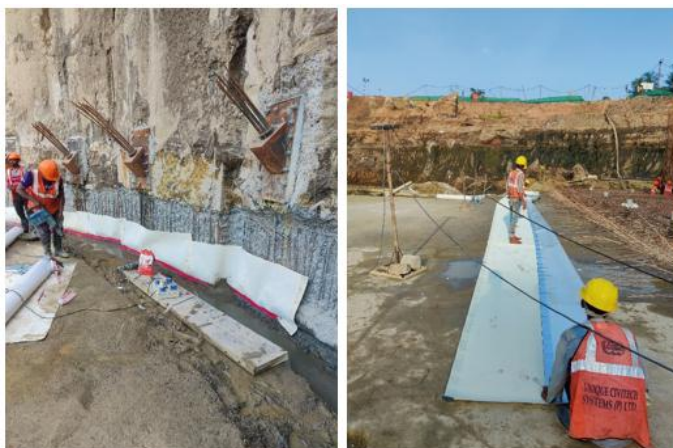
(Fig 8.HDPE - waterproofing membrane installation)
