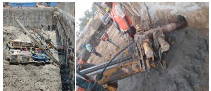
(Fig 7. Diaphragm wall anchoring process)
