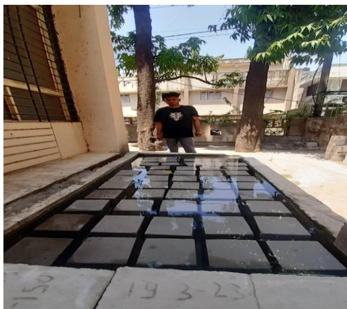
Fig-1: Concrete Curing
