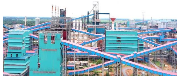
Figure 3 Raw material junction houses
