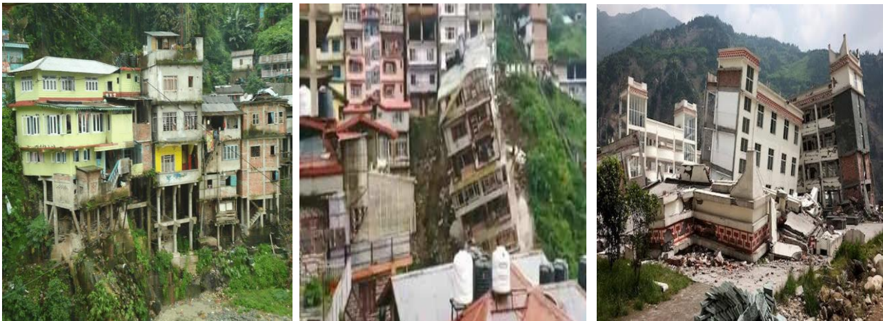
Fig. 1. Damage and collapse of multi-story buildings due to major earthquake in hilly areas.
