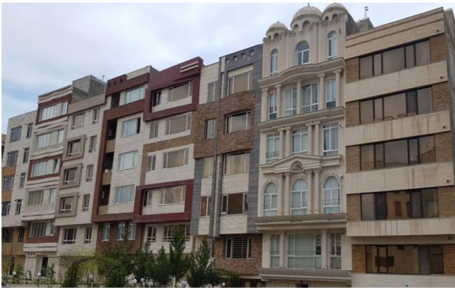
Fig -1: Adjacent Buildings in Tehran with different floor heights & without separation gap between them
