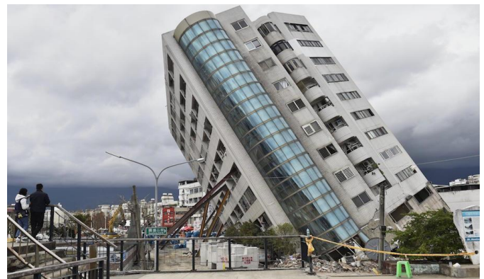
Fig.1: Collapsed Building Due to Earthquake
