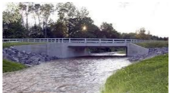
Figure 5 RCC Solid Slab Culvert
