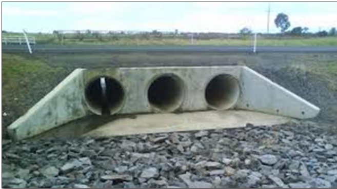
Figure 2. Three Cell Pipe Culvert
