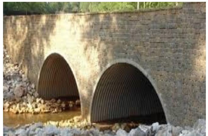
Figure 4 Arch Type Pipe Culvert
