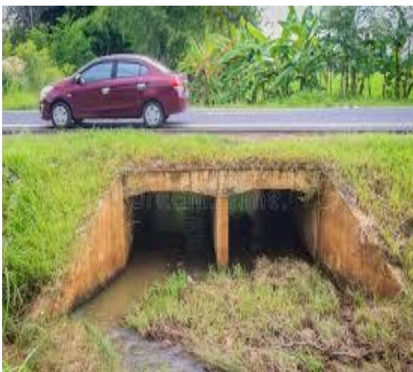
Figure 3 Two Cell Box Culvert
