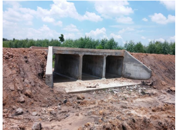
Figure 1-3 cell Box Culvert
