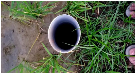
Fig 2.1 Installation of Pani pipe
