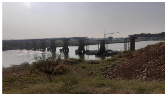
Bridge under construction site for case study
