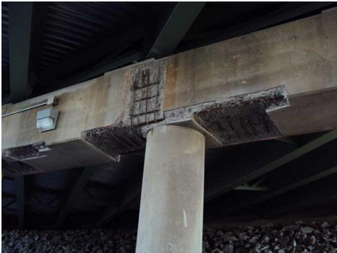
Figure-3: Jacketing of the Bridge.
