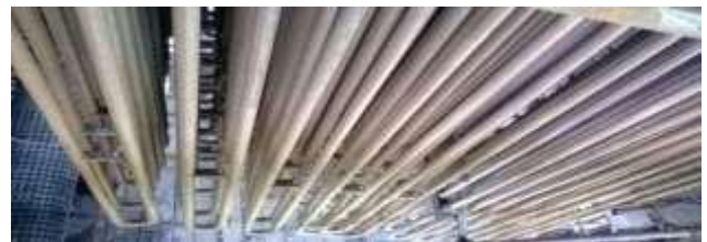
Fig.1.2 Actual photograph Super heater tubes of a boiler
