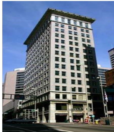
Figure-01: First RC Frame Structure (Skyscraper)
