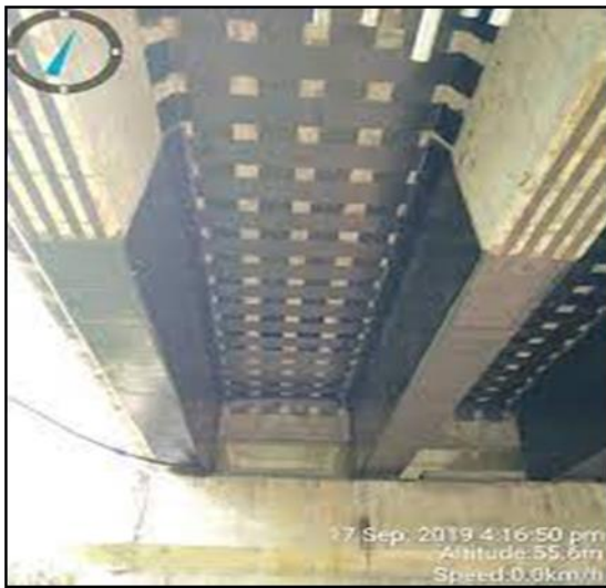
Fig 1:- FRP jacketing of Bridge deck from bottom
