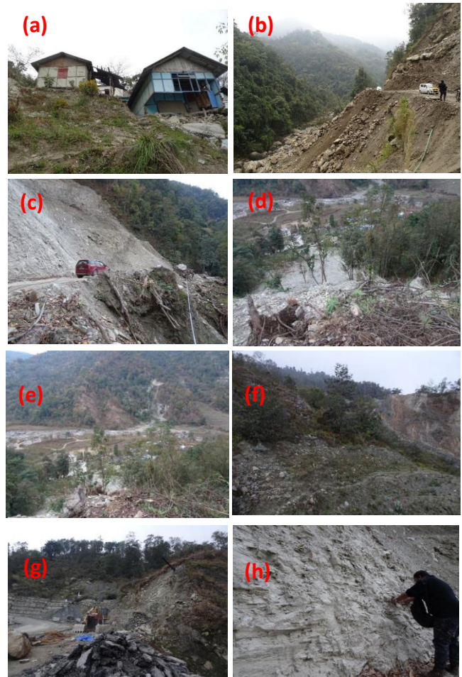
Fig -5: Photographs during field investigation (a) Affected houses due to Pachey Slide (b) debris flow at Qu Khola Slide (c) Teen taal Slide (d) Devasted vegetation (e) Vulnerable settlements in the Valley (f) Kit Golai Slide (g)Vulnerable road construction (h) Fragile lithology.
