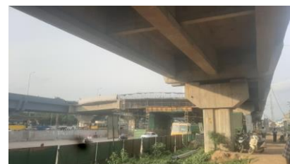
Fig 5: Perungalathur bridge under construction
