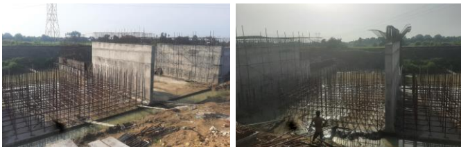
Fig 7: Minor bridge at Vembakkam
