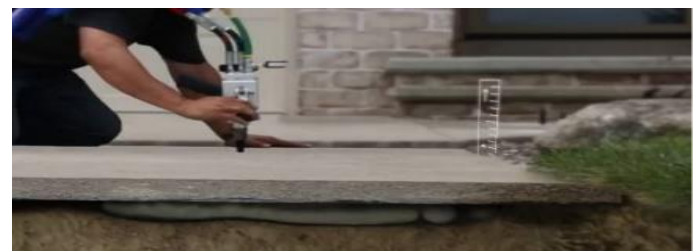
Fig. 2.7: Polyurethane Foam for BPM.
