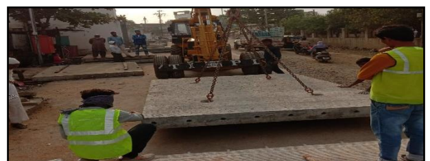
Fig.1.4: Placing of Panels.
