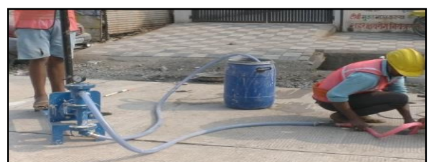
Fig.1.5: Grouting of Panels
