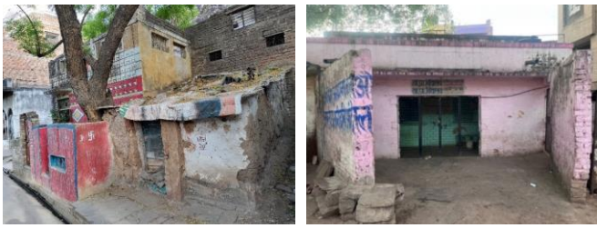
Fig -12: House Conditions and School in Lakshmanpura Slum, Gwalior
