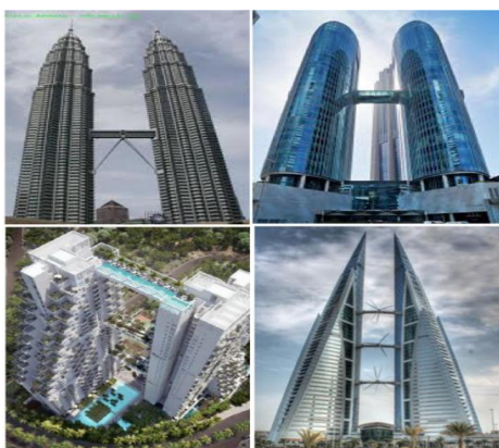
Fig -6: Horizontal Walk Connected Building
