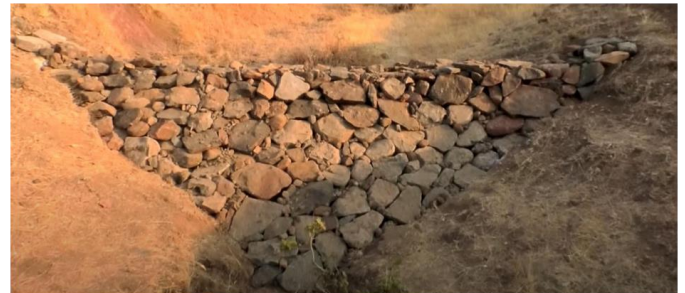
Fig -1: Loose Boulder Structure
