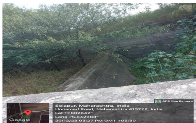
Fig - 6: Check Dam at Darfal
