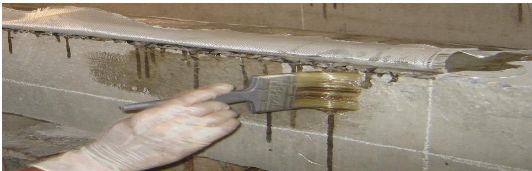
Fig. 3.10 Application of Epoxy and Hardener on the Beam
