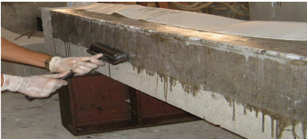
Fig. 3.12 Roller used for Removal of Air Bubbles
