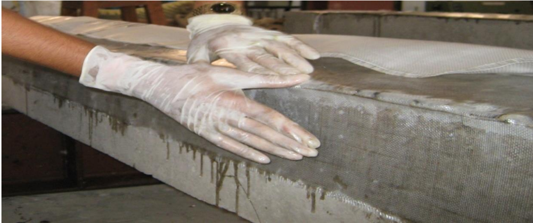
Fig. 3.11 Fixing of GFRP sheet on the beam
