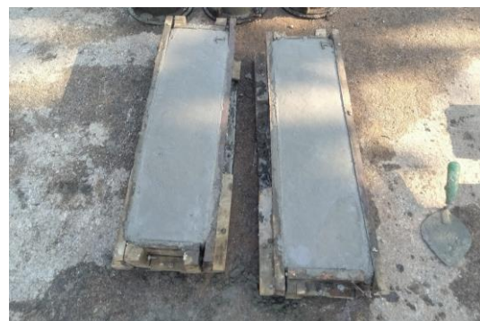
Fig-3: Casting of Beam
