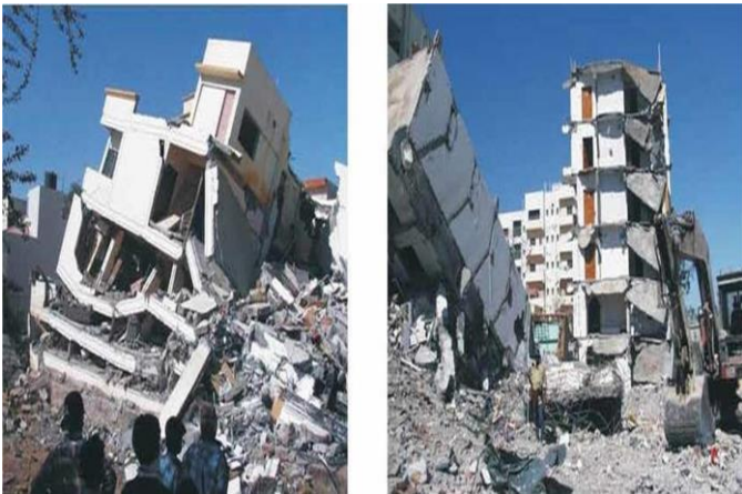
Figure 1 Failure in the 2001 Bhuj earthquake
