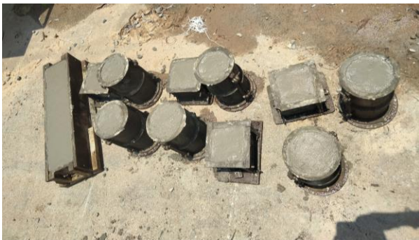
Fig-1: - Casting of Cubes, Beam & Cylinders.
