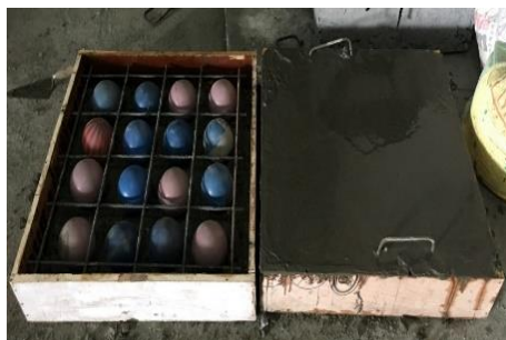
Fig.9 Using 90mm Balls and placed for casting in a Grid form
