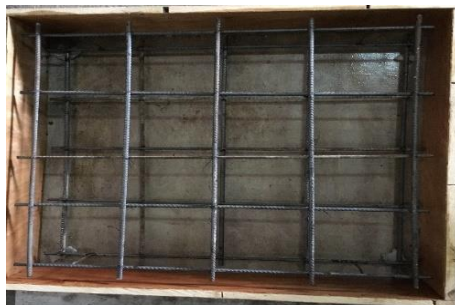
Fig.8 Fe 500 Bar 10mm Dia @ 240mm Spacing from Centre to Centre in 0.7m X 0.7m X 0.15m Mould
