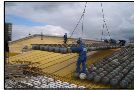
Fig.2. Casting Bubbles on Building
