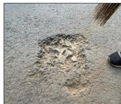
Fig- 7: Cleaning the Pothole
