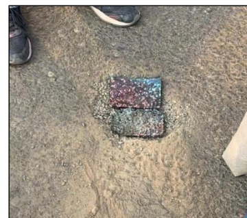
Fig- 9: Placing the HDPE Plate
