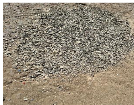
Fig-14: Pothole filled on 28th January 2023
