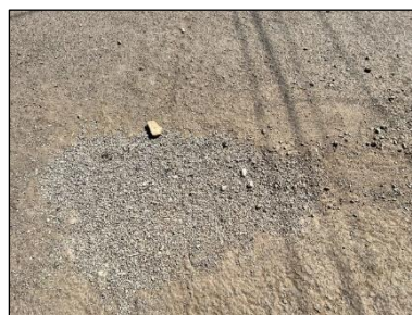
Fig- 12: Filled Pothole with HDPE Plate
