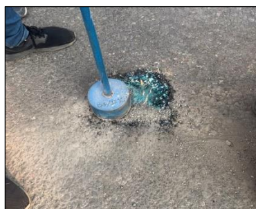
Fig- 11: Compaction with Rammer
