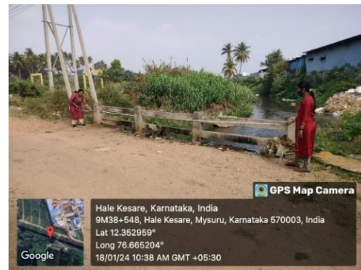
Plate - 2: Measurement of Width of Drain
