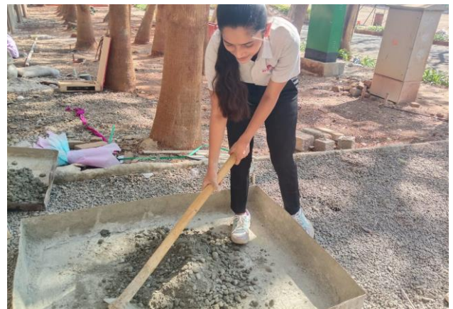
FIG.No. 3.5. MIXING OF CONCRETE
