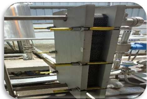
Fig.1 Plate Type Heat Exchanger
