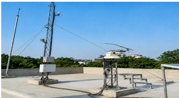
Figure 4. Setup installed by NIWE.
