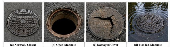
Fig.3. Representative manhole conditions considered for monitoring.
