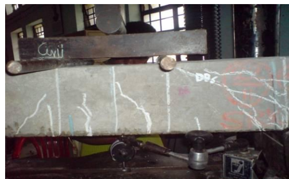
Fig.11 Shear and flexural cracks
