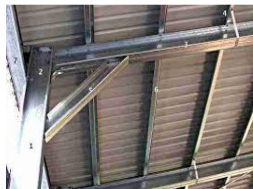
Fig -1: Knee bracing
