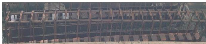
Fig-11: Reinforcement cage for composite beam with Type 2 shear connector ready for casting
