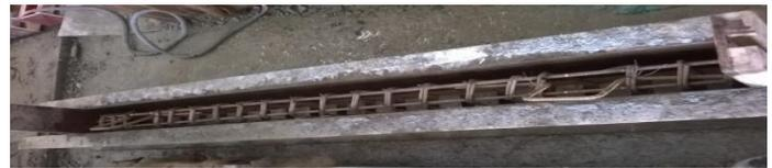
Fig-13: Moulds with reinforcement cages ready for casting
