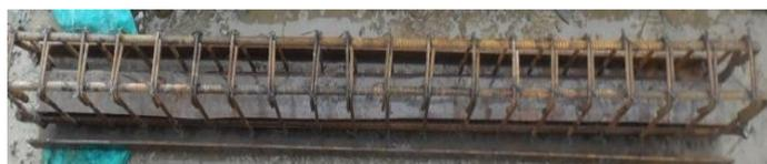
Fig-12: Reinforcement cage for composite beam with Type 3 shear connector ready for casting
