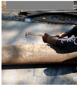
Figure B- General Setup of conventional gas cutting of pipe
