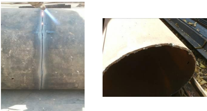
Figure D- Side and front view of MS pipe during and after cutting
