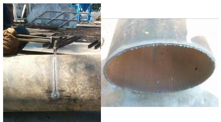
Figure C- View of pipe during and post cutting
