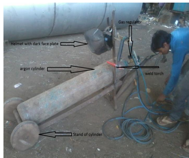
Figure 2. GTAW set up (Courtesy: Apex Engineering, Dediyaan, GIDC-II, Mehana)
