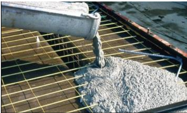
Fig -4.4(c): Pouring of RMC
