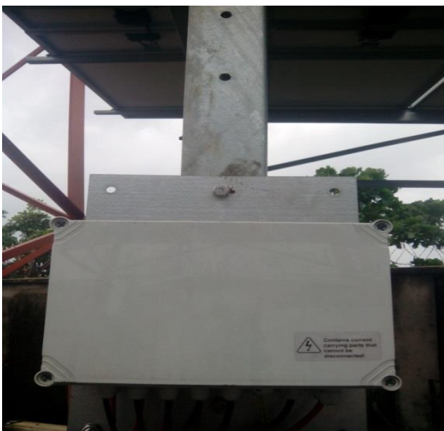
Fig-11: Solar Panels
