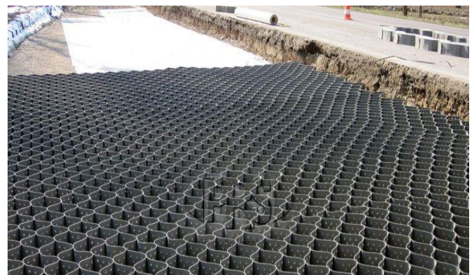
Fig-6: Geocell geotextile for road construction [22]
