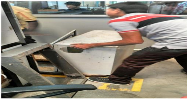
Fig 5.8: Moving away unwanted materials and panels
