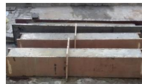
Fig 6:- Concrete surface is smoothed
