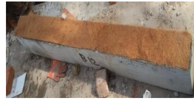
Fig10:- Beams wrapped with RCF sheets
