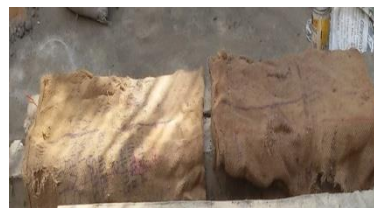
Fig 8:- Curing of beams
