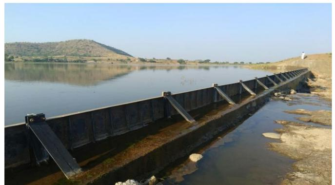
Figure-10: Water storage created by Needle Type Gates at Virkhel M.I. Tank, Taluka Sakri, District Dhule.
