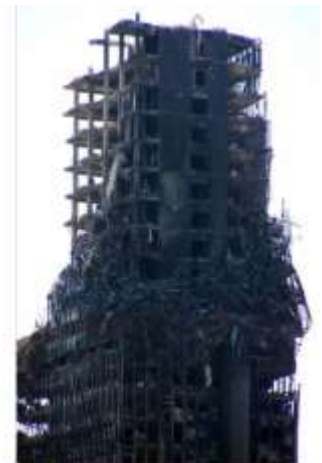
Fig.1.2 Windsor Tower After Fire
