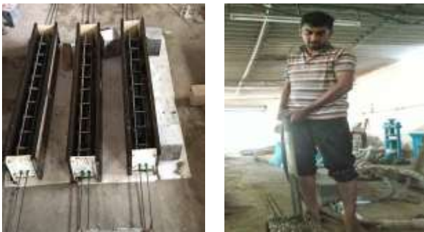
Fig 2:- Casting of Post Tensioned Beams
