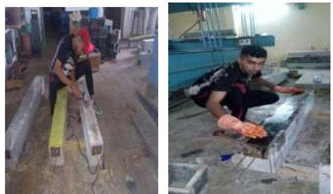
Fig 4:-Leveling and Application of epoxy and CFRP Laminate
