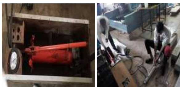
Fig 3:- Post-tensioning of beams
