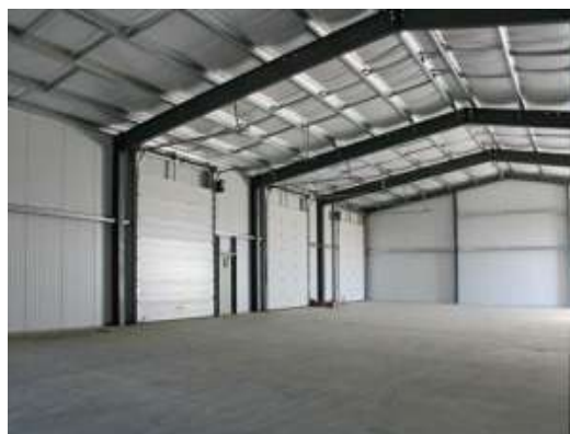
Fig 1. Rigid frame structure
