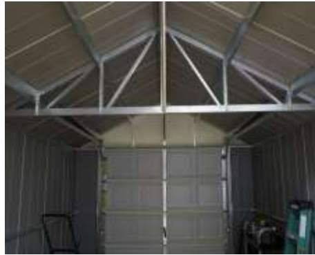
Fig 2. Steel truss structure
