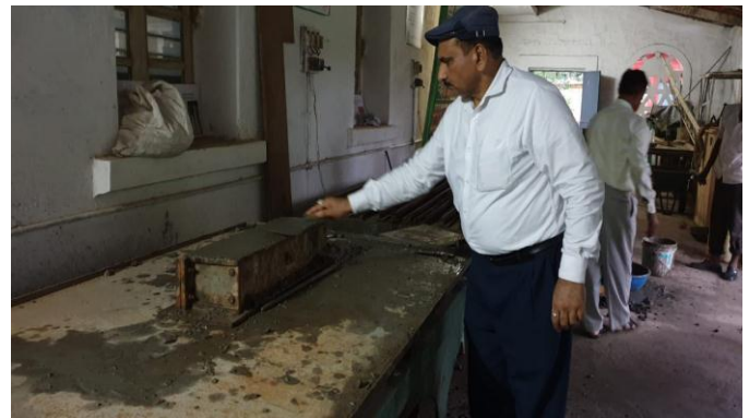
Figure: 2.6 Casting of moulds of Beams.
