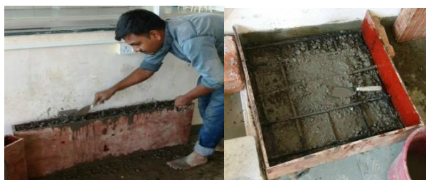
Fig no:5 casting of wall
