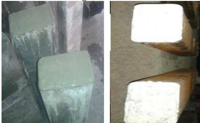
Fig 2.3.1 CASTING of CFST columns
