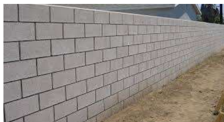
Fig -3: Hollow Concrete Blocks Construction
